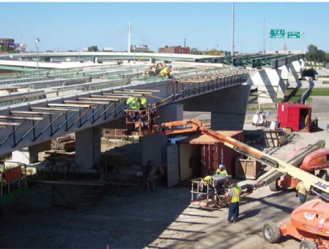
View of on-going work on SO2 ramp
