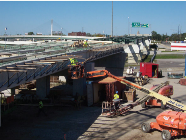
View of DIBC (white) and MDOT (green) portions of SO2 ramp
