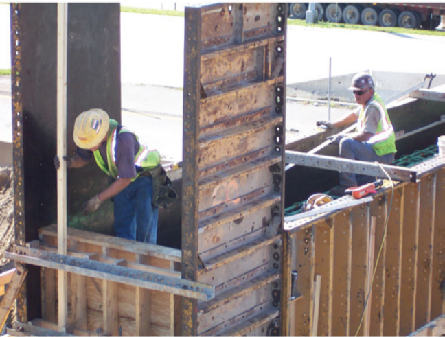
Local contractors working on pier cap form
