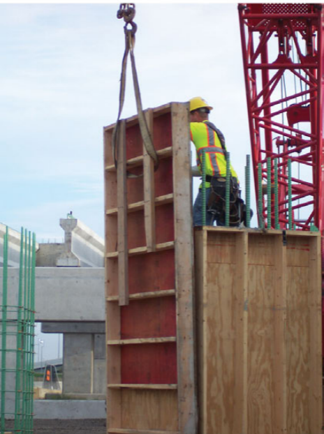
Workers removing frame after concrete has cured
