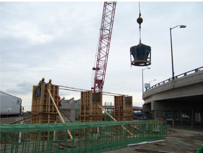
Concrete transport to location to pour
