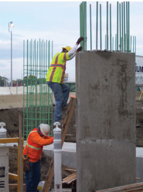
Wood frame removed exposing cured concrete column
