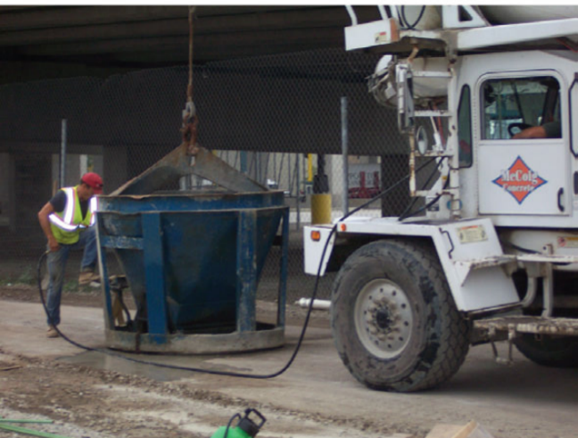
Concrete ready to transport
