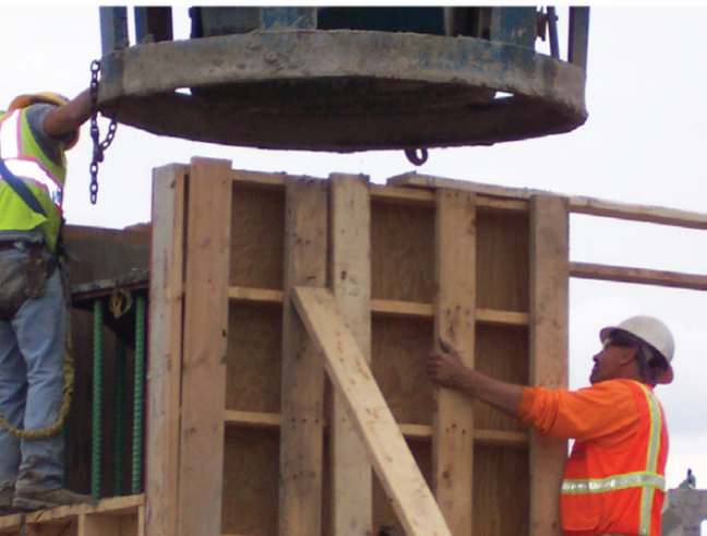
Ready to drop concrete into column form
