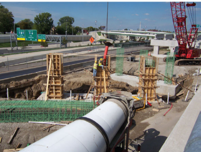
Prepping columns prior to pouring concrete
