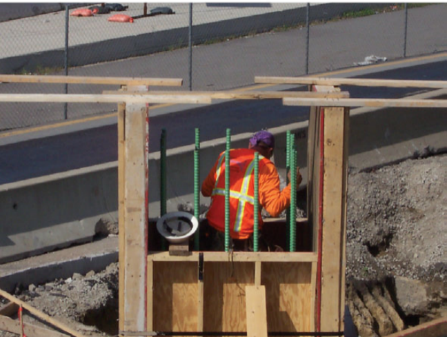
Worker prepping column of pier
