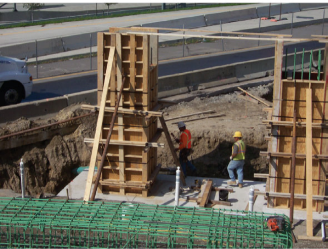
Prepping columns prior to pouring concrete
