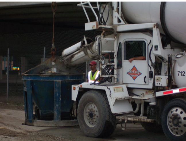
Concrete being poured into cylinder for transport
