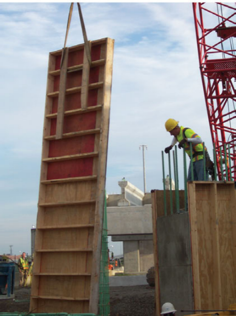
Workers removing frame after concrete has cured
