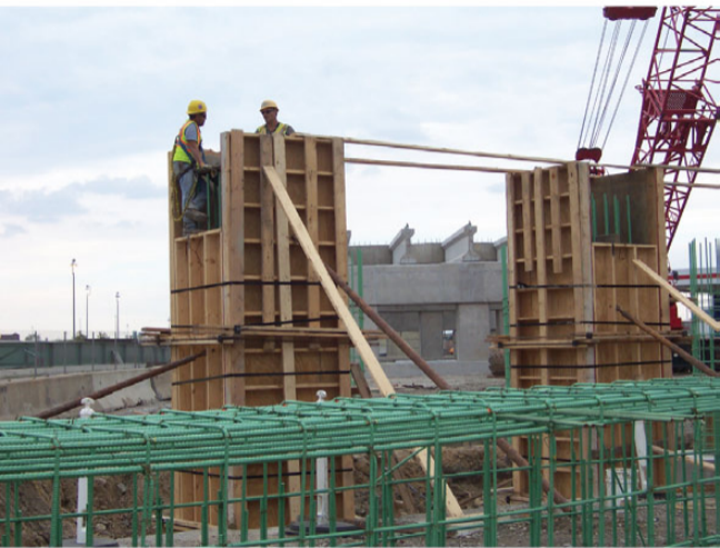
Getting ready to remove frame for one of the columns
