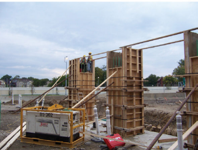
Getting ready to remove frame for one of the columns
