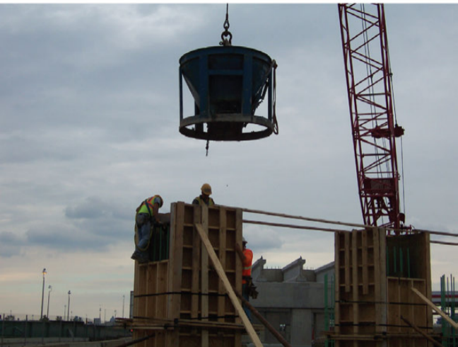
Ready to drop concrete into column form
