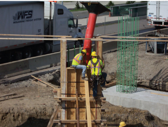
Closer view - Lowering steel support beam before pouring concrete for pier
