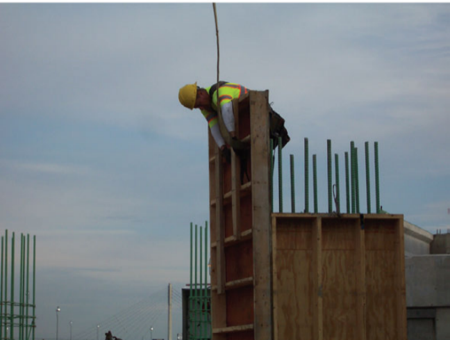
Workers removing frame after concrete has cured
