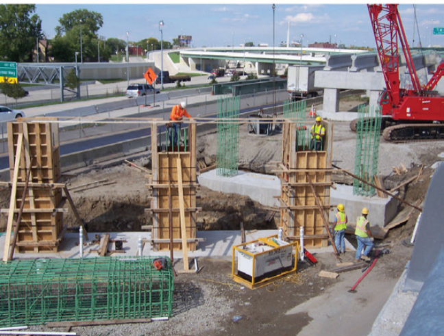
Prepping columns prior to pouring concrete
