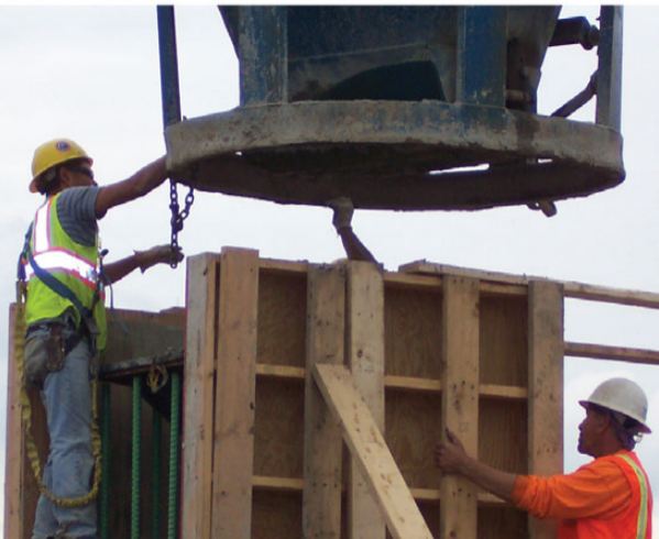
Ready to drop concrete into column form
